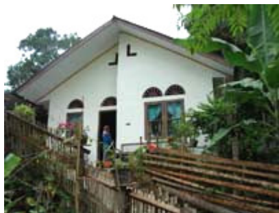
One of the 2500 houses completed out of the 3800 to be built.
